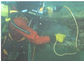
Figure 2 – Ultrasonic test of steel member by diver in UK
